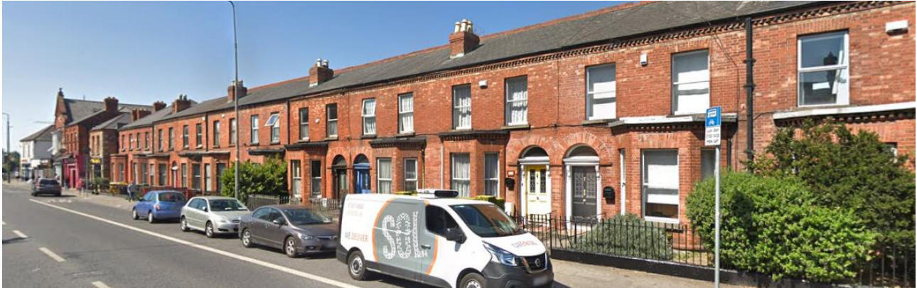
FIGURE 11 EXISTING TERRACED HOUSING ON THE SOUTH CIRCULAR ROAD
